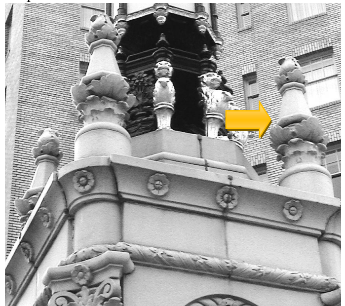
Figure 1: Replacement finial (right) 20 years after casting using Custom System 45 mixed with Restoration Latex RL-2.
