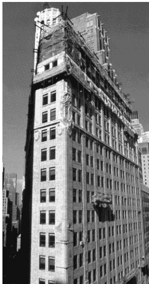
Figure 3 (left): Pump-X53 was used to fill voids between terra cotta band courses and rubble masonry backup on this project in New York City. Figure 4 (right): Injection points are marked on an interior wall surface; Pump-X53i was injected through the back-up wall into the masonry exterior veneer to fill cracks and voids in the stonework.
