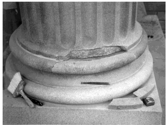
Figure 5: Column base, before/after bonding with Flexi-Weld 520T .
