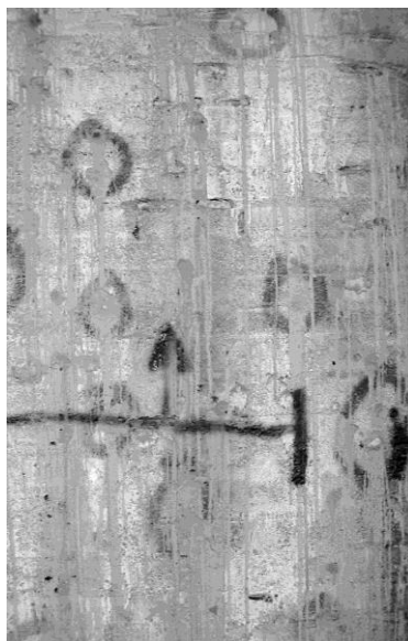
Figure 3 (left): Pump-X53 was used to fill voids between terra cotta band courses and rubble masonry backup on this project in New York City. Figure 4 (right): Injection points are marked on an interior wall surface; Pump-X53i was injected through the back-up wall into the masonry exterior veneer to fill cracks and voids in the stonework.
