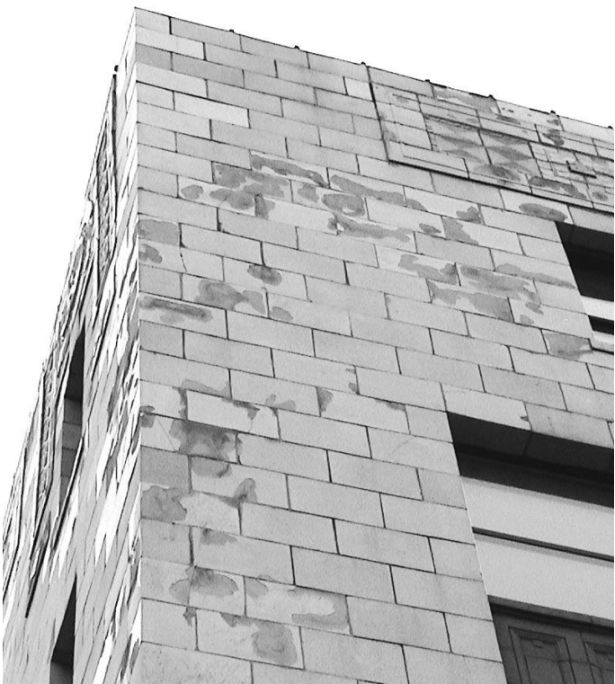
Figure 2: Thin-Section glaze spalls are common in terra cotta subjected to bulk moisture infiltration.
