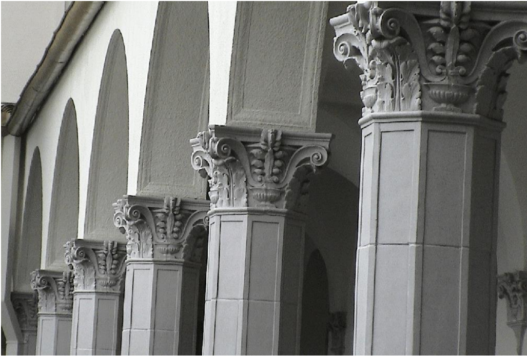
Completed sections of replacement castings are shown above.
