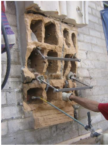
Figure 1. Failed Terra Cotta Bracket, 230 Park Avenue
