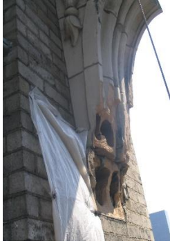
Figure 1. Failed Terra Cotta Bracket, 230 Park Avenue
