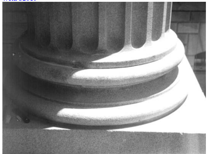
Figure 5: Stone column base, before and after rebonding with Flexi-Weld 520T .
