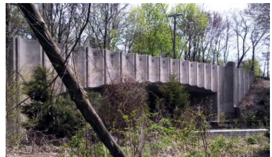
Photo: The Madison Avenue Bridge on Connecticut's National Landmark Merritt Parkway had repair sections repoured using REPLIC-8 , custom-matched by Edison Coatings, Inc..
