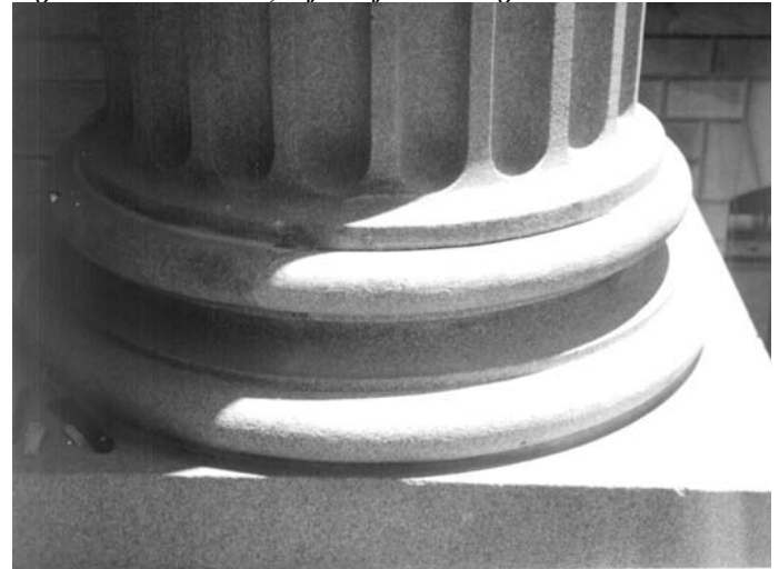
Figure 5: Column base, before/after bonding with Flexi-Weld 520T .
