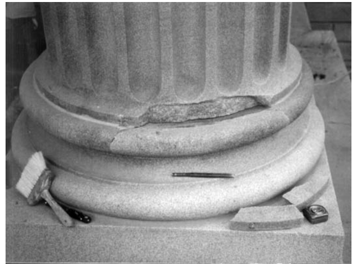
Figure 5: Column base, before/after bonding with Flexi-Weld 520T .
