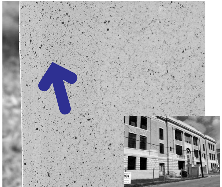
Where's the Repair? Glazed terra cotta spall, upper left corner, filled and smoothed using Thin-Fill 55 prior to glazing and speckling with Aquathane UA210 coatings, matched to original glaze colors. Project is an Historic school restoration in Charleston, SC.
