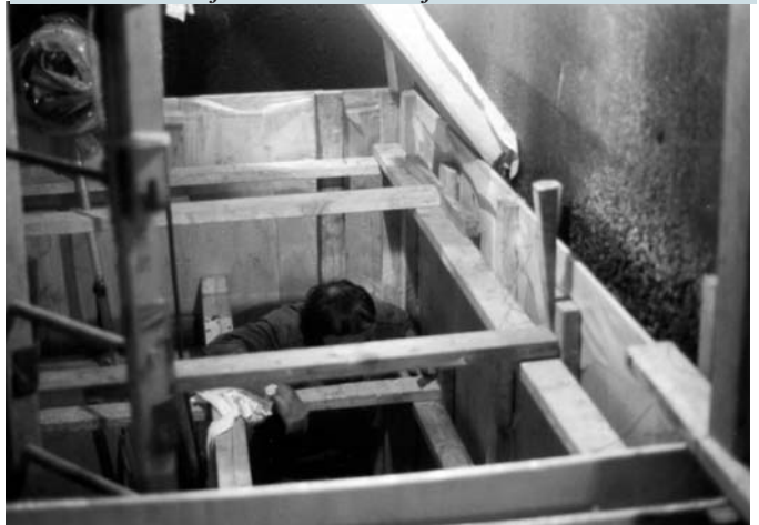
PHOTOS: FLEXI-MATRIX 545 flows down a polyethylene-lined chute into a plywood form. The walls of this chemical wastewater sump were eroded to depths up to 9 inches. Following construction of a new reinforcing steel grid, and using the eroded wall as the rear of the form, plywood forms were set and a new, structurally independent polymer concrete tank was poured. Wall thickness ranged from 6 to 15 inches. Height was 8 feet. The final stages of pouring and set occurred after the tank was refilled with wastewater.
